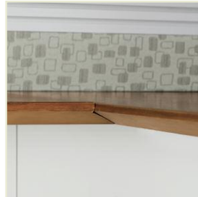
Coped edge on connecting worksurfaces
